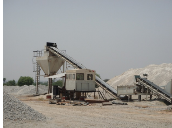
Image: Aggregate Crusher
