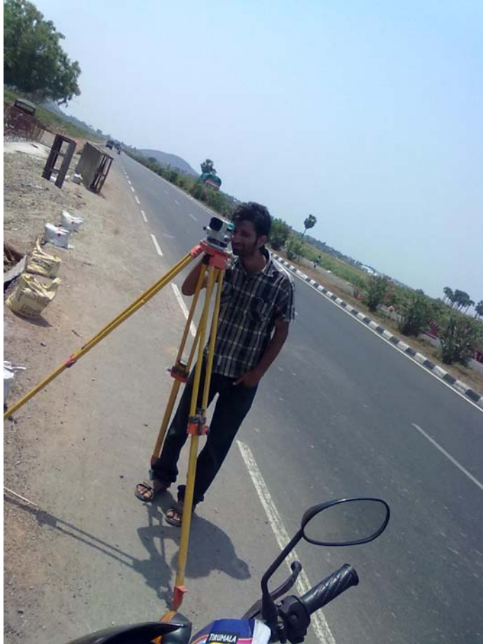
Surveying using dumpy level
