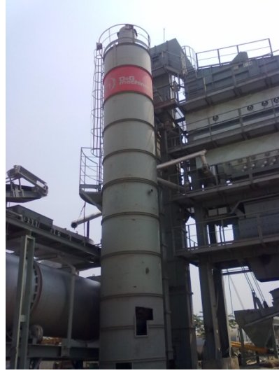
Image: Single barrel Asphalt Premix Plant.
