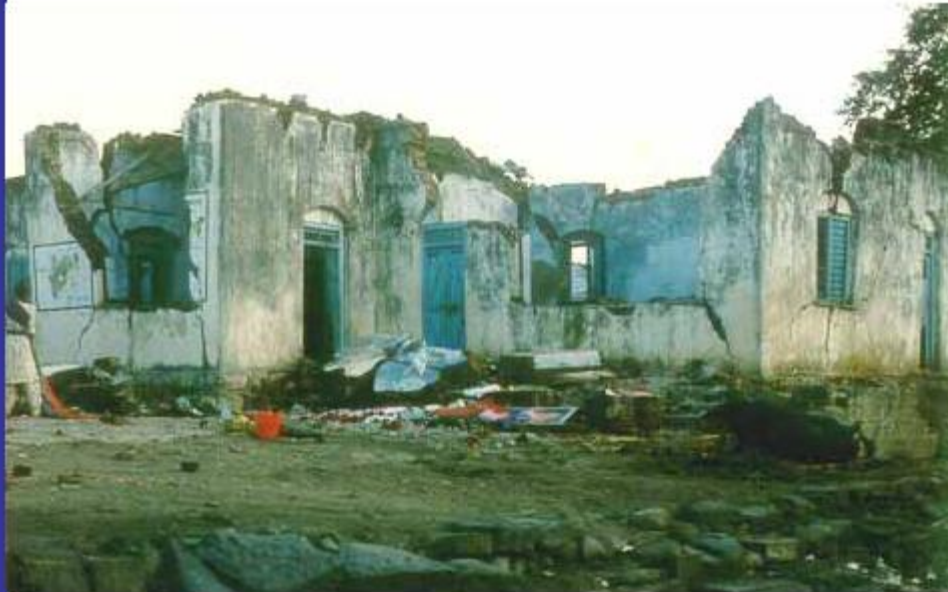
(a) Building with no horizontal lintel band: collapse of roof and walls
