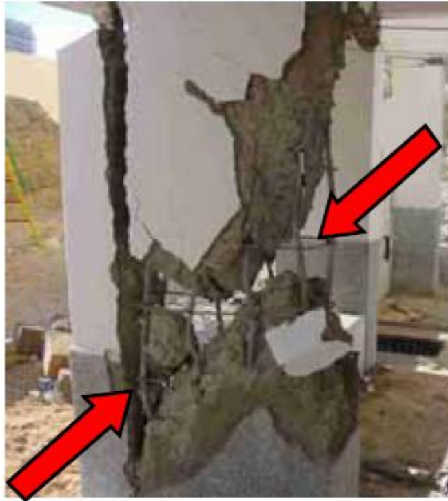
Figure 2: Diagonal cracks in columns jeopardize vertical load carrying capacity of buildings - unacceptable damage.
