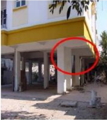
Damage to buildings with offsets
