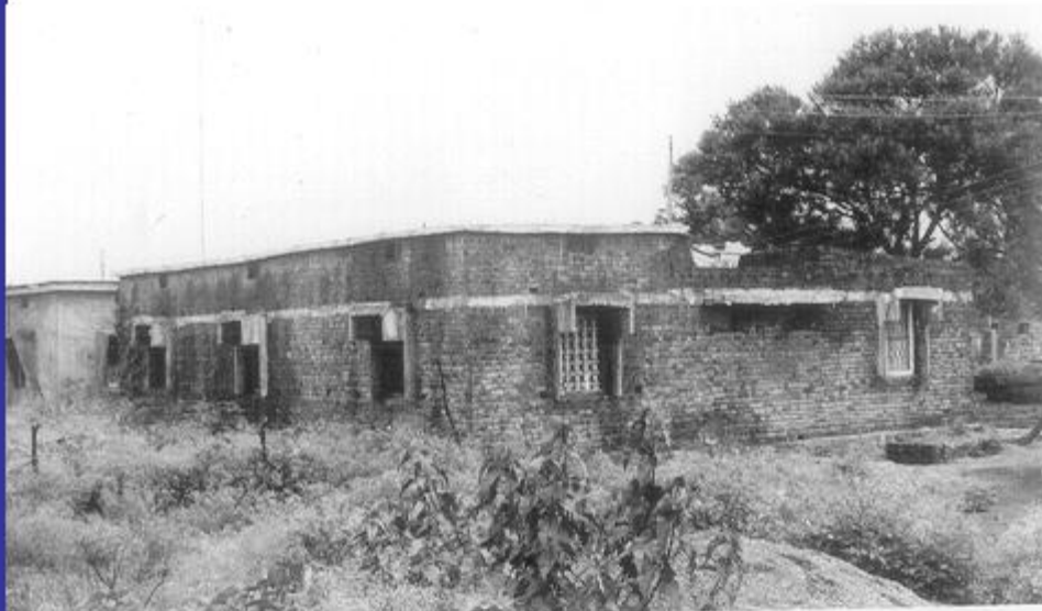
(b) A building with horizontal lintel band in Killari village: no damage
