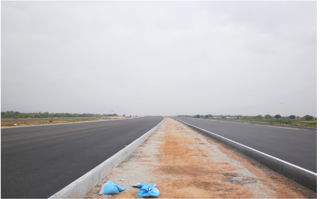
A view of DENSE BITUMINOUS MACADAM
