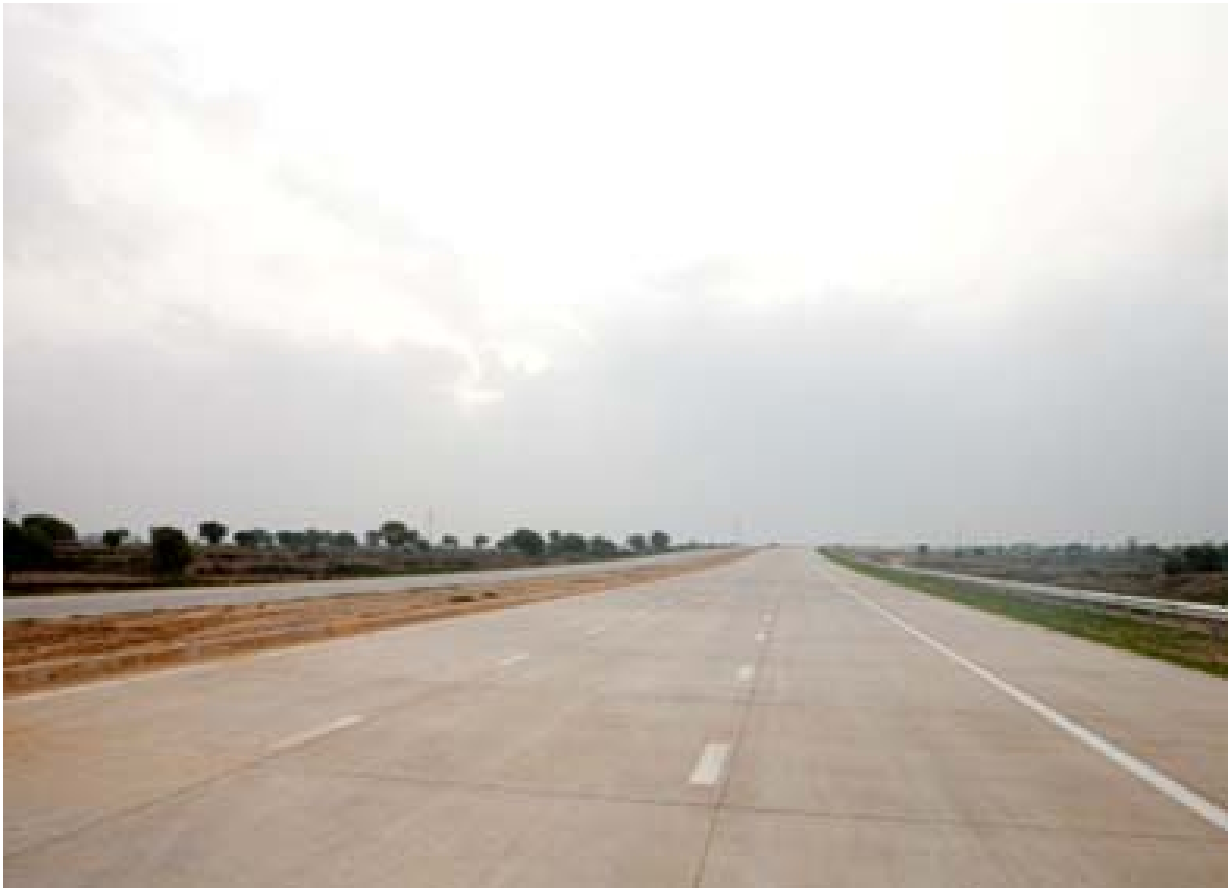
Fig 2: A view of rigid pavement
