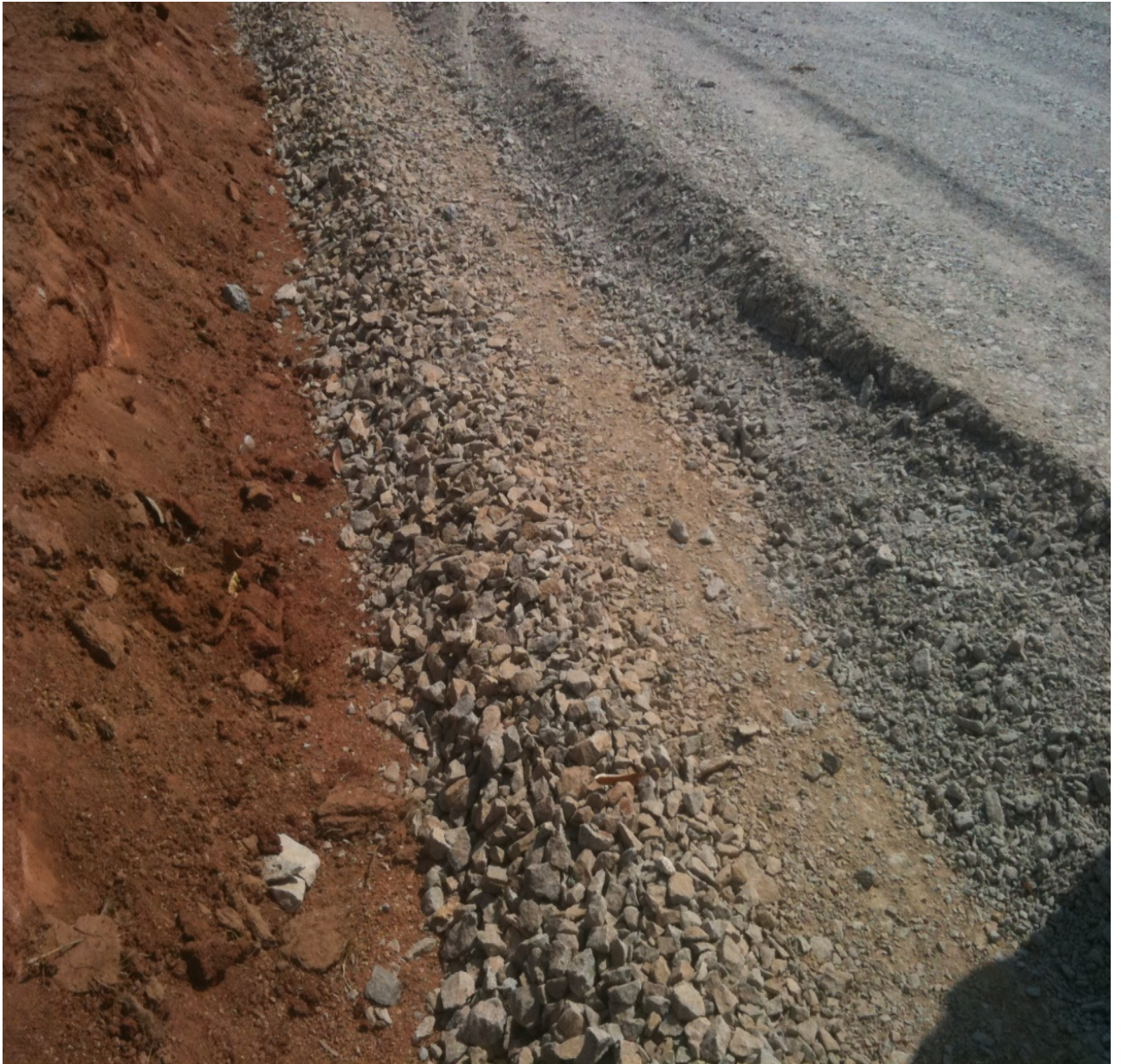
Fig 1: A view of Flexible pavement components
