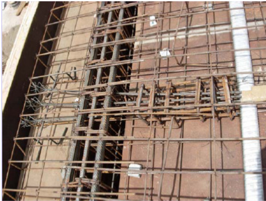
Figure 9. Anchorage by looping the wires in a Slab.
