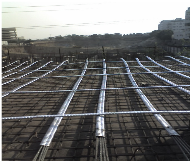
Figure 19. Tendon arrangement.
