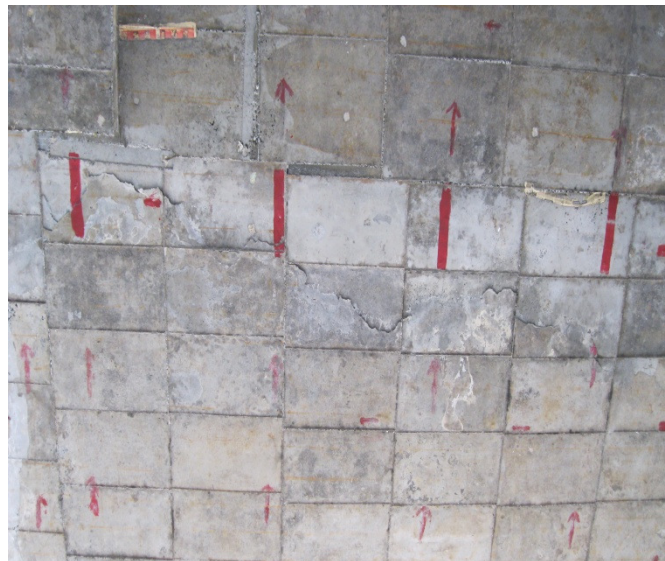
Figure 39: Soffit marking used to indicate tendon position & arrangement..
