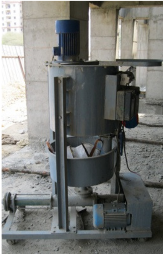
Figure 15. Grout mixer and pump
