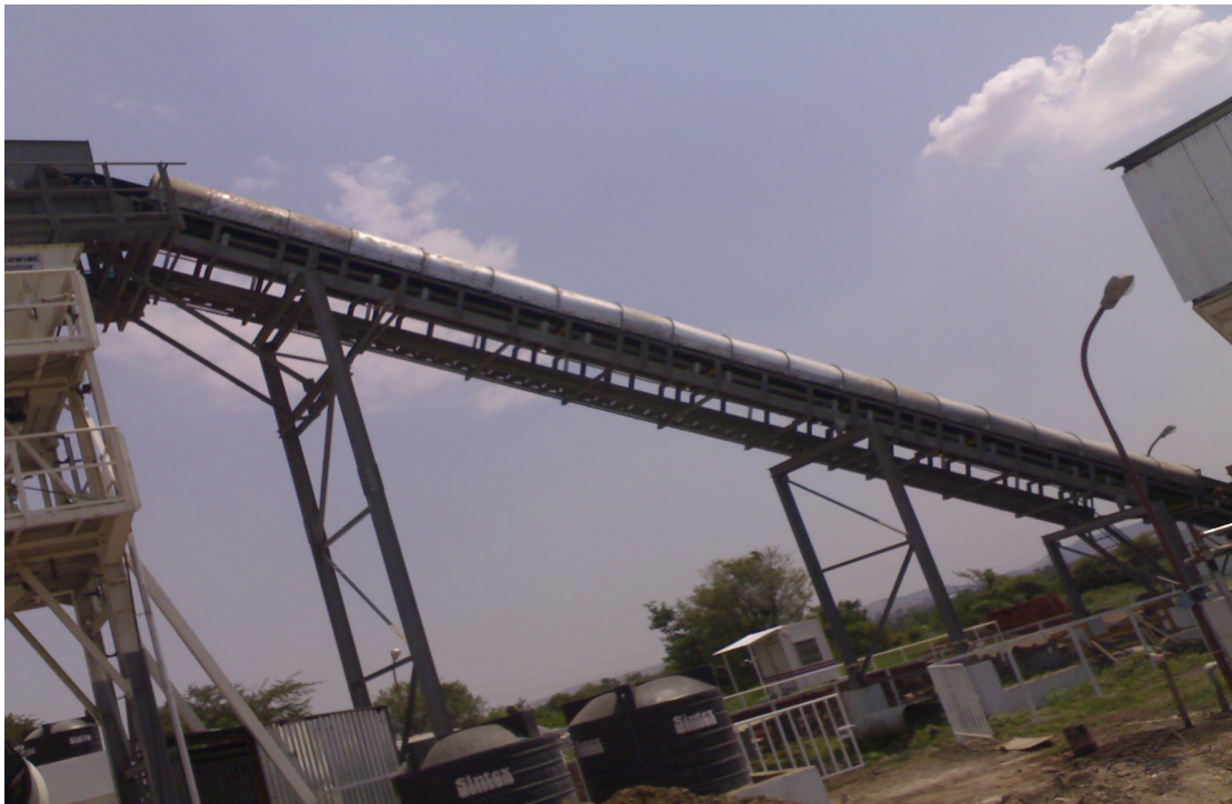
Belt conveyer (To feed Raw material to the holding hopper)
