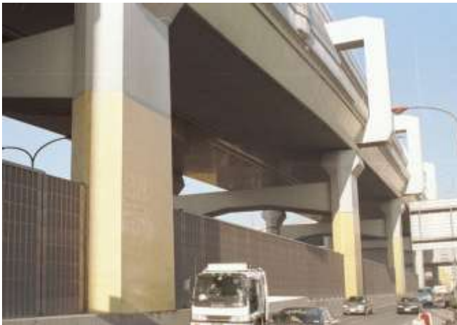
Strengthening for bridge piers
