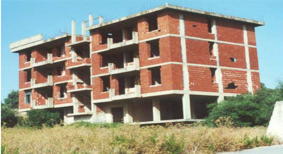
Fig. 15 Building owned by IACP of Syracuse in the village of Solarino
