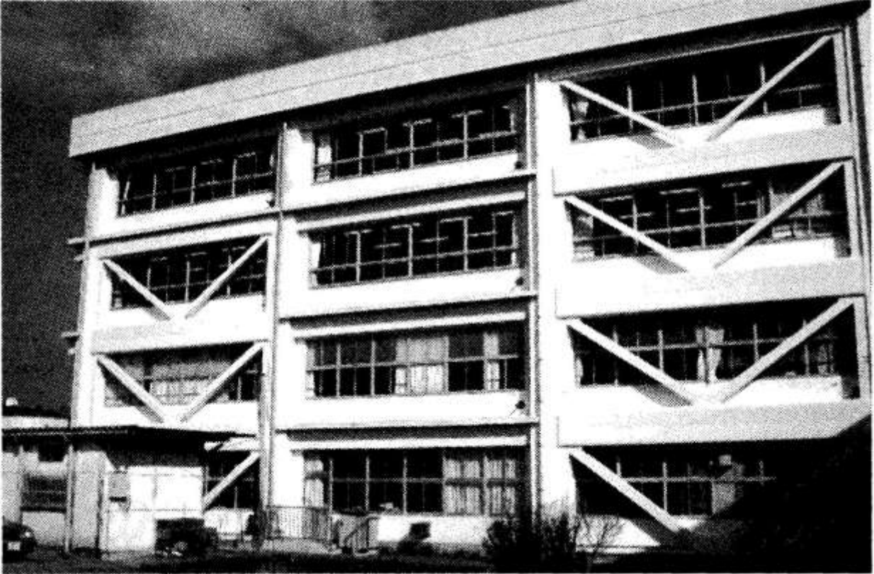
Retrofitted school building
