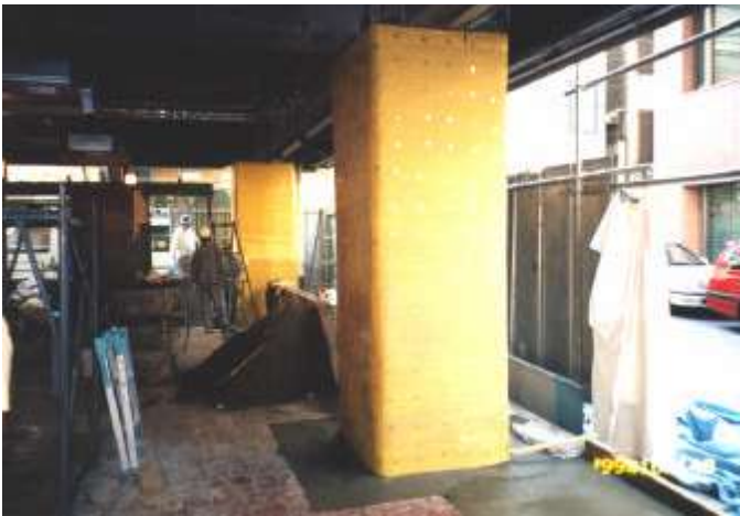
Shear strengthening of building columns
