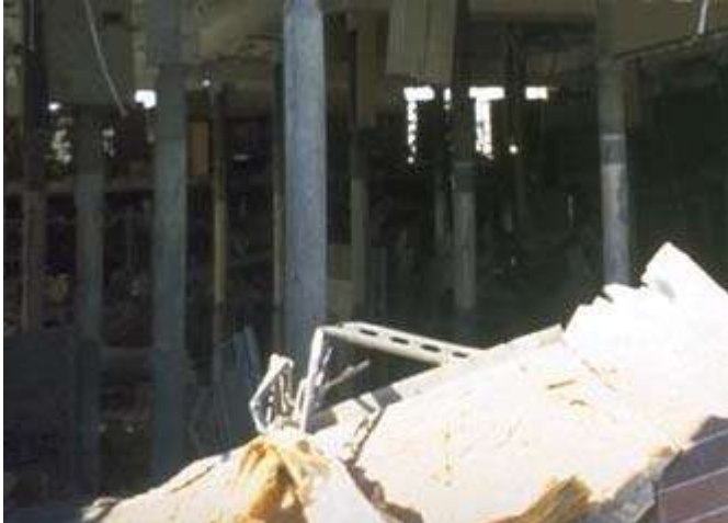
Slab-column connection failure – Northridge earthquake
