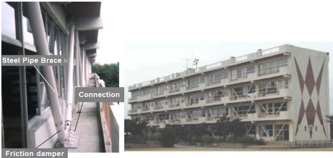
Photo. 4 Application to a balconied school building
