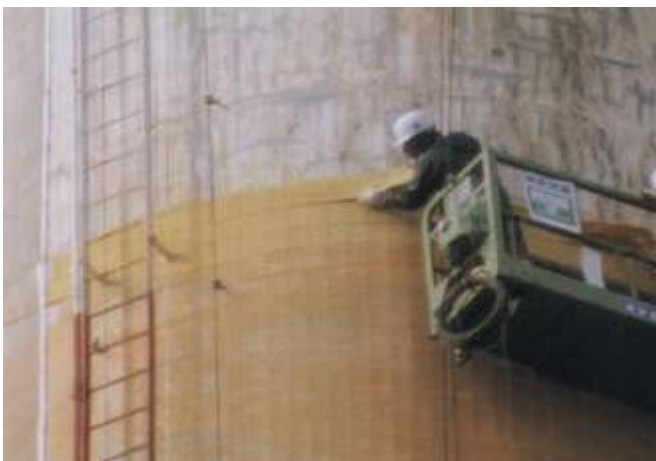
Repair for chimney
