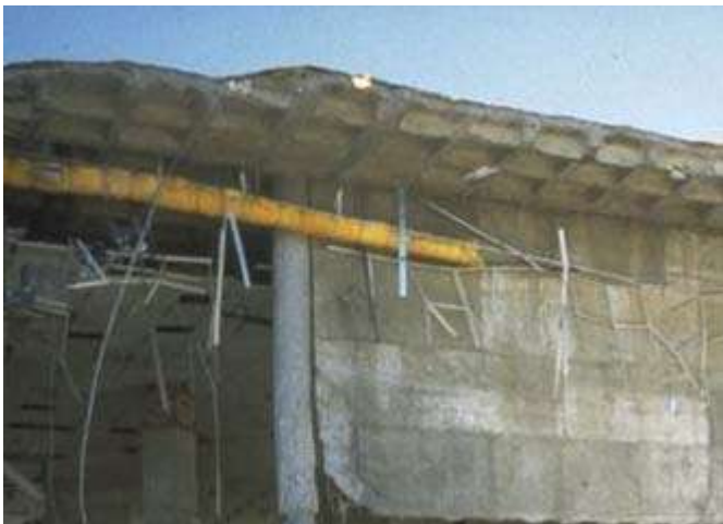
Joint failures – Northridge earthquake
