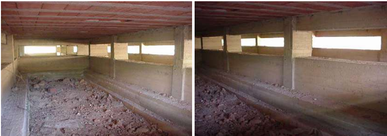
Fig. 16 Foundations of an IACP building in Solarino
