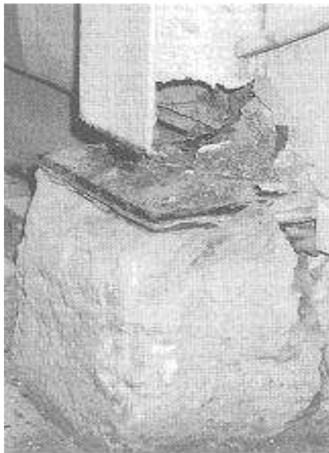
Fig. 2 Deteriorated Column Base
