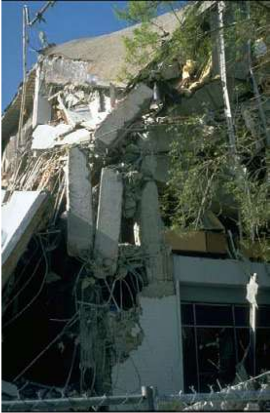
Joint failures – Northridge earthquake
