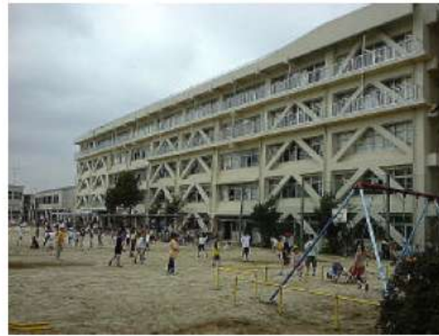
d) Elementary School Building (with Balconies)
